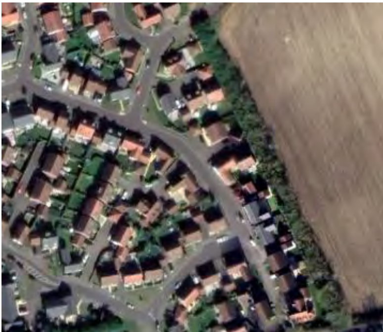
Aldridge Way, in the north eastern part of the town (see Photograph 46) - development (again including some 2½ storey properties) again extends right up to the edge of the settlement.
